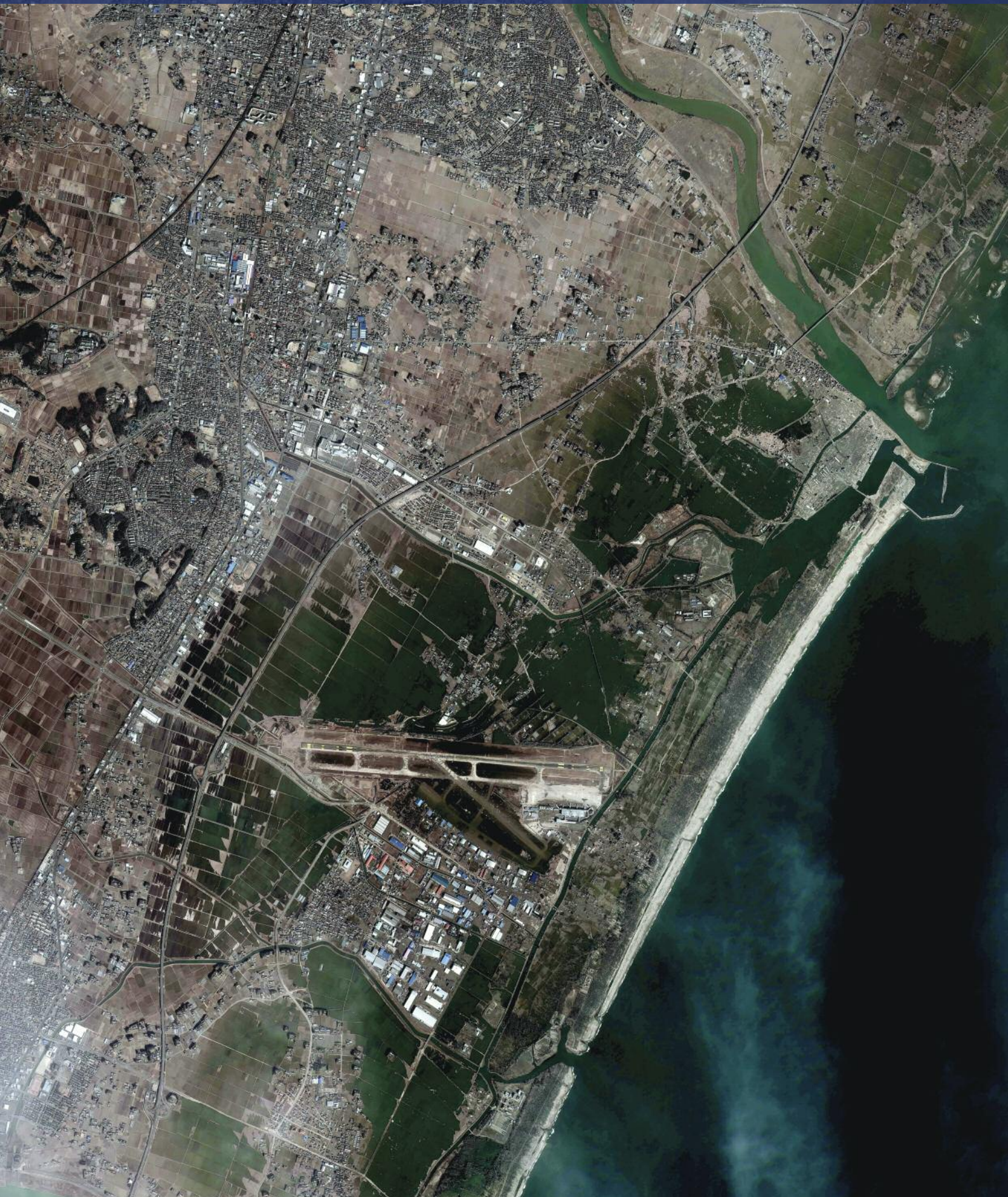
Tsunami damaged area observed by KOMPSAT-2 on 14 March 2011 over Sendai, Japan after an earthquake and tsunami struck the region. The destroyed infrastructure, debris and flooded area are visible in this image.
